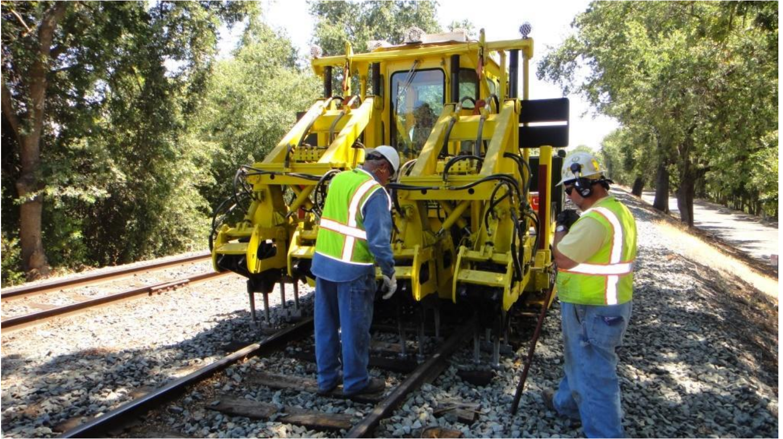
Scott guides the tamper as Mike F. prepares to remove jacks
