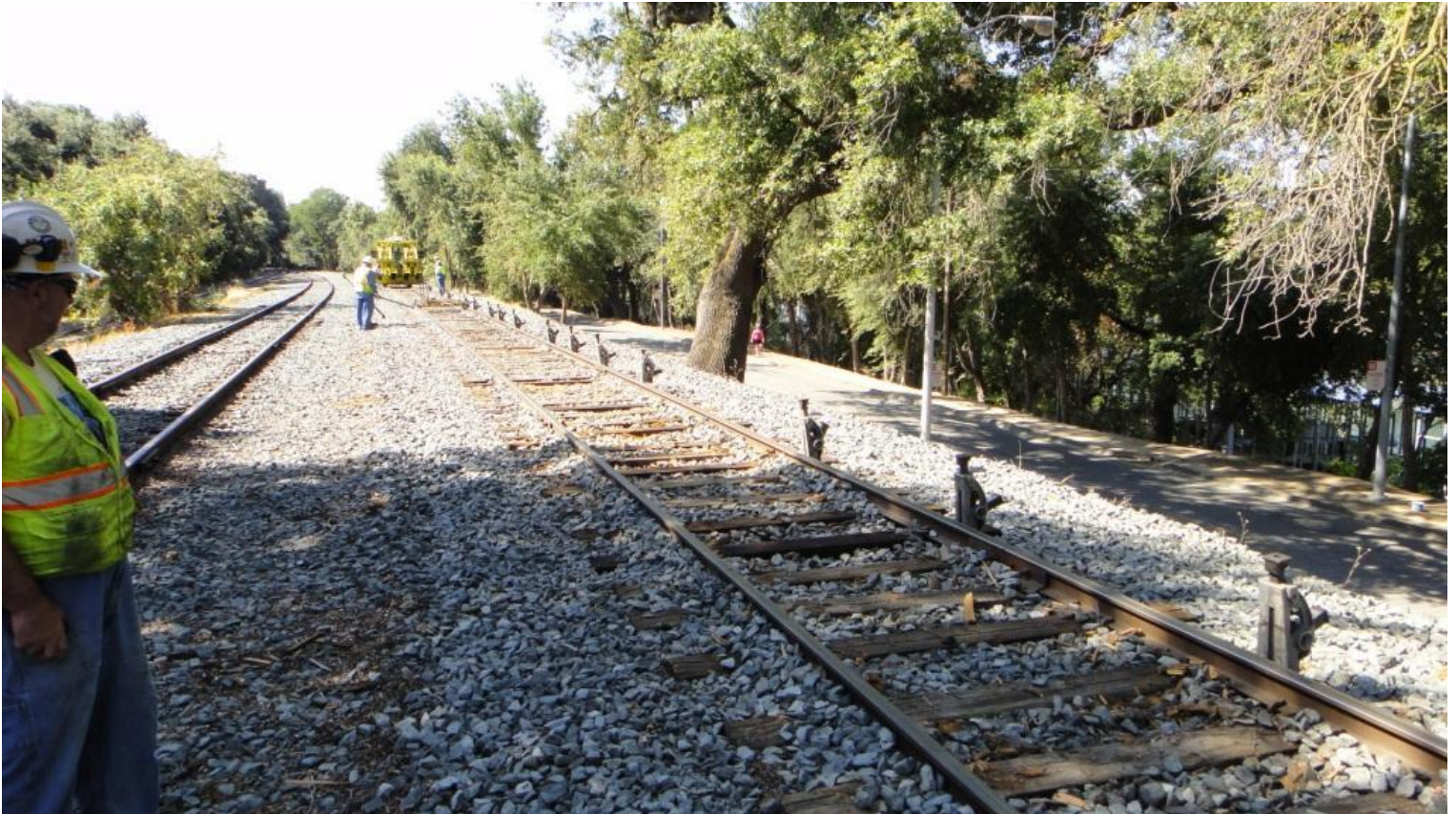
With jacks in place, the track is level. Time to bring in the tamper
