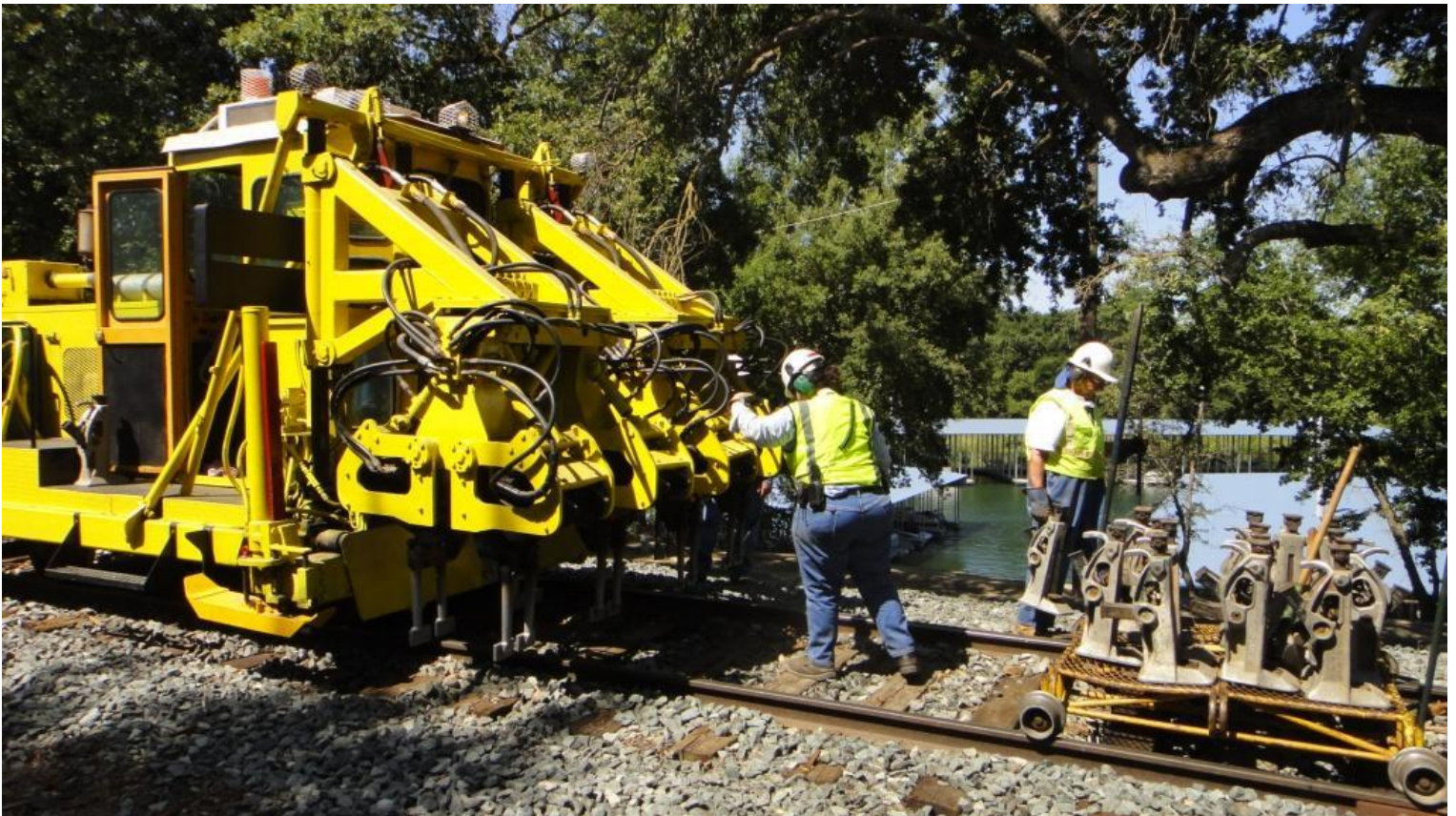
Heather guides Chris in the tamper as Clem loads jacks onto the Nolan Track Cart
