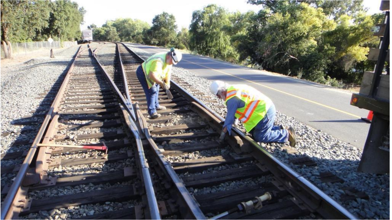
Frank W. and Frank S. installing gauge-rods between the frog and guard-rail at Switch 17
