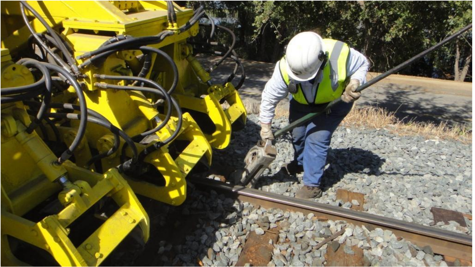
As the tamper comes in, Heather removes a jack
