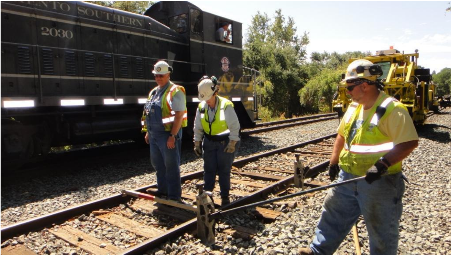
The 11 o'clock train passes by while Chris and Heather verify the level as Mike F. lifts the west rail with the track-jack
