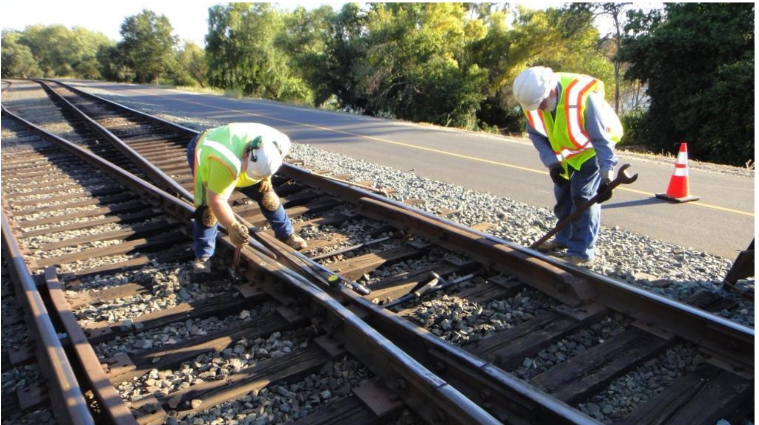
Frank W. and Frank S. use crescent and track-wrenches to tighten-down the gauge-rods
